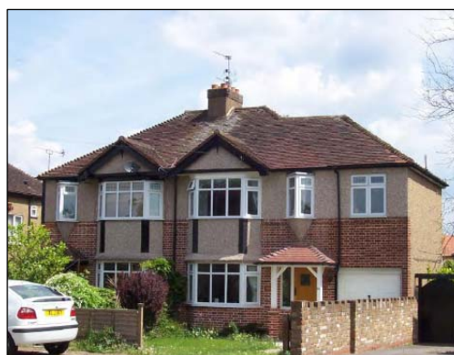
Example of a well designed side extension
