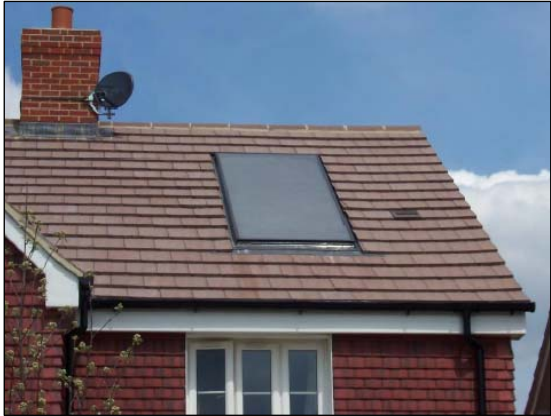
Flush mounted solar panels
