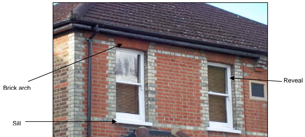
Diagram 9: Components of a window and opening
