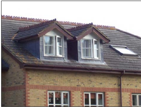
Dormers aligning with windows below and roof form and detail to match existing roof
