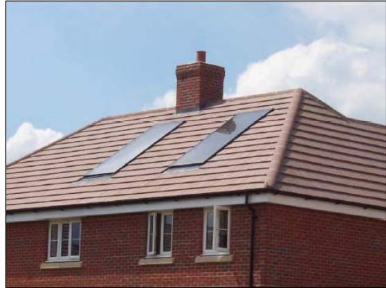
Flush mounted solar panels
