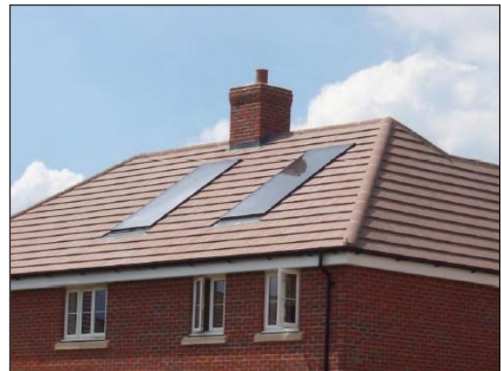
Flush mounted solar panels
