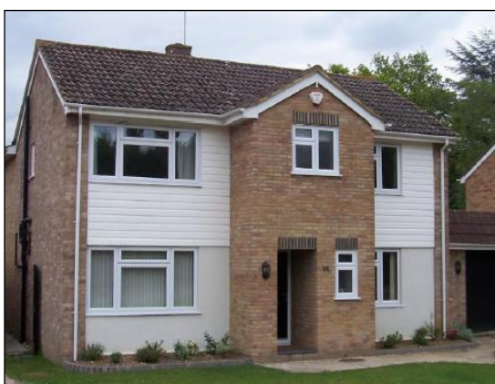
Balanced front extension to a detached property
