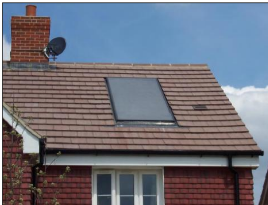
Flush mounted solar panels
