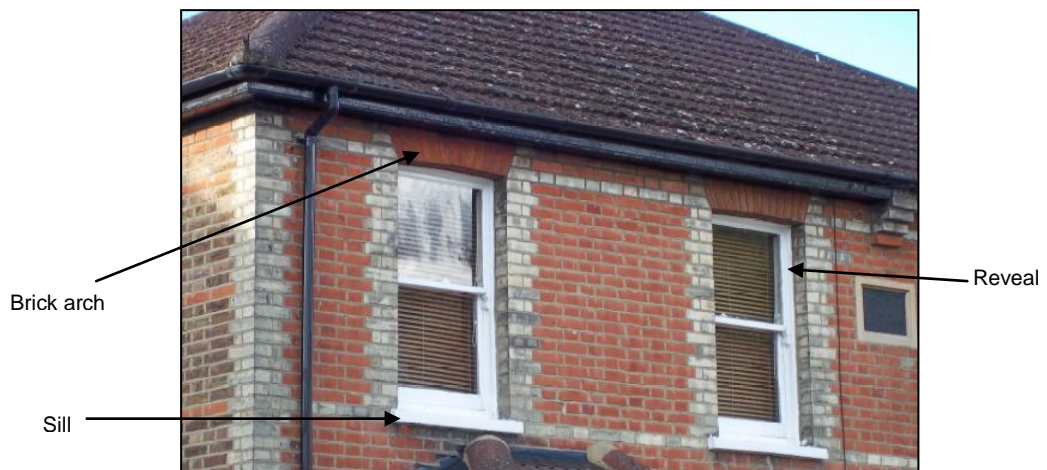
Diagram 9: Components of a window and opening
