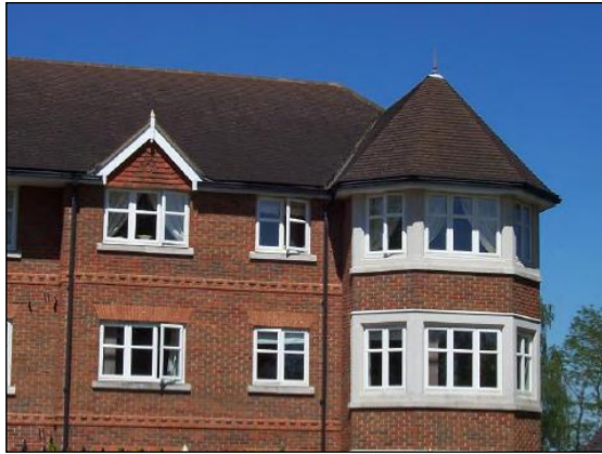
Roof, brick and stone detailing
