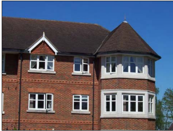
Roof, brick and stone detailing
