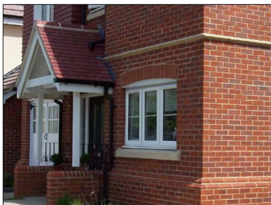
Brick and stone detailing
