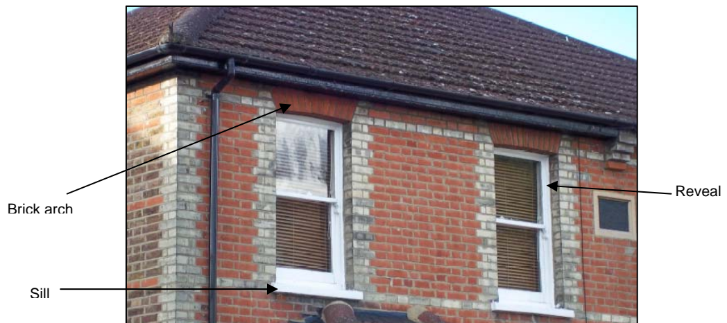
Diagram 9: Components of a window and opening
