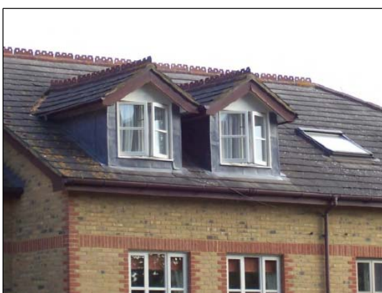
Dormers aligning with windows below and roof form and detail to match existing roof
