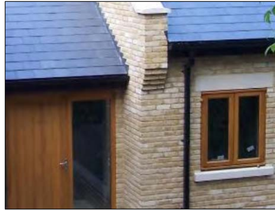
Brick, stone and lead detailing
