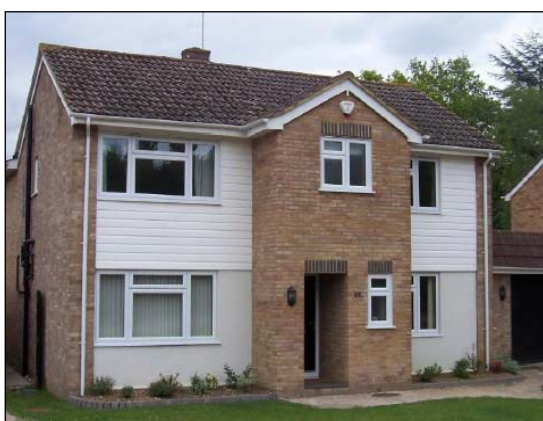
Balanced front extension to a detached property
