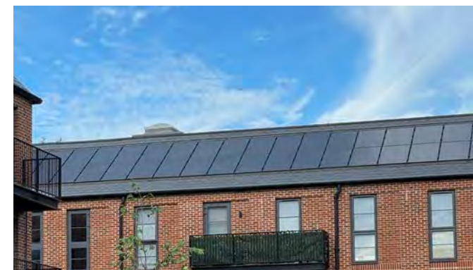
Flush photovoltaic panels incorporated into a roof
