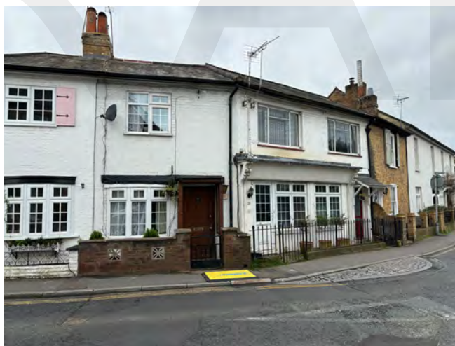
Historic properties at the south of the character area, adjacent to the historic core. Note the redundant fascia board which denotes a former shopfront, since lost.
