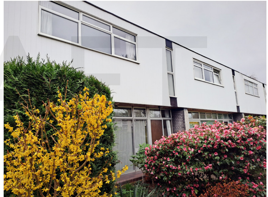
Modernist terraces in phase 2. Note the horizontally-configured windows and projecting upper storey.
