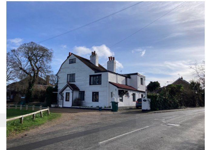
This building constitutes two cottages, the oldest phase to the left having been first built as a barn in 1720. Its irregular roofline, timber weatherboarding and windows of mixed styles and proportions identify it as a vernacular structure. The partial survival of the barn, incorporated into a later dwelling house, evidences the agricultural economy which sustained Lower Halliford for most of its history.
