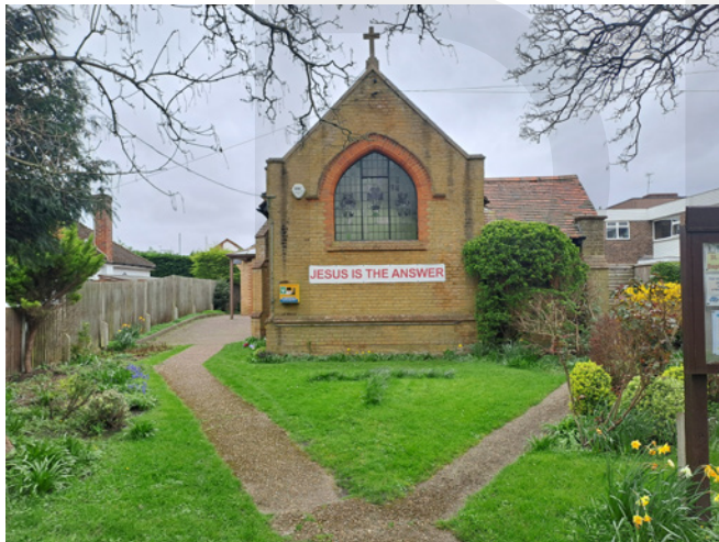
St Andrews Church, constructed in 1900, utilised a traditional materiality of exposed red and yellow brick.
