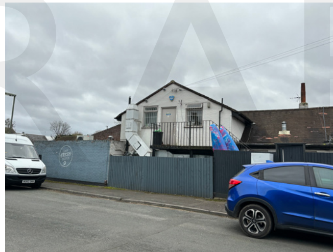
Visually prominent servicing and inappropriate timber fenced boundary treatment to the Goat Inn.
