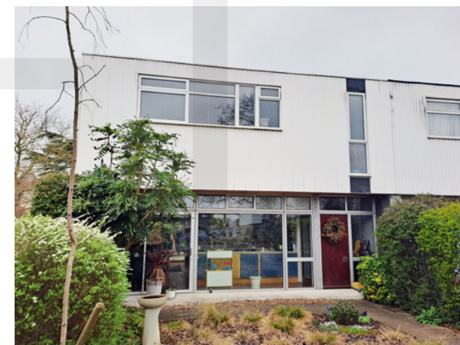
Original full-height glazing to the ground floor on an east-facing elevation in phase 1. The original plain door, faced with plywood, has been retained in-situ.
