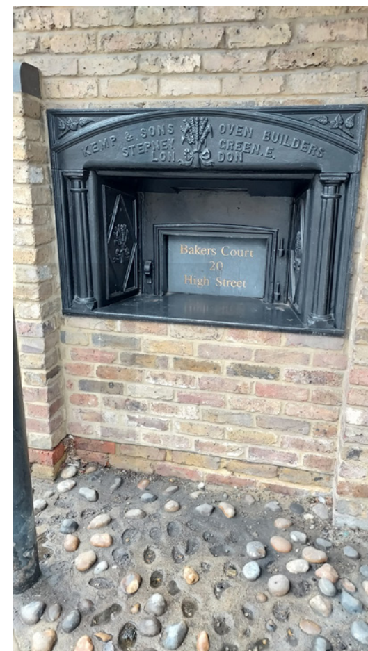
A retained section of a cast iron oven at 20 High Street.
