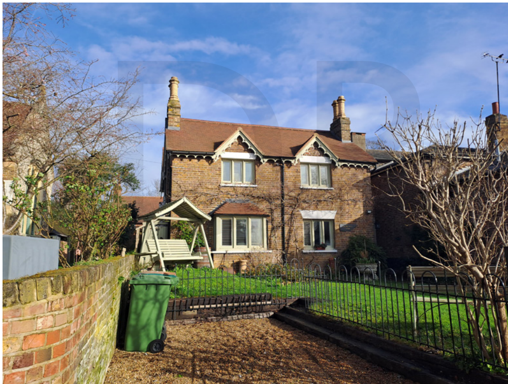
Old Ferry Cottage, Ferry Square. The scalloped bargeboards and tall patterned chimney pots are vernacular inspired features.
