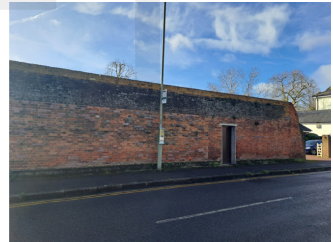
An example of a high brick boundary wall on the south side of Chertsey Road.
