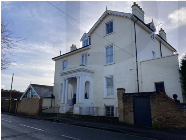
The regular fenestration and grand doric portico at Mill Eyot are typical Neo-Classical features. The wavy-edged bargeboards and finials are however more reminiscent of the 19th-century Gothic revival. Mill Eyot was built in the mid-19th century when Gothic was beginning to eclipse Neo-Classical as the dominant architectural style.
