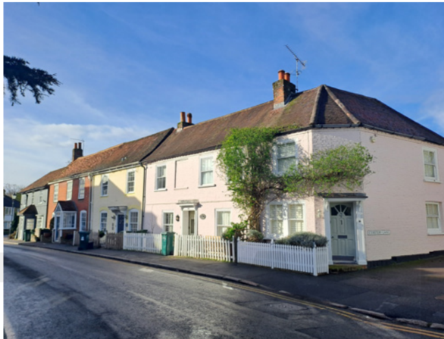
A terrace of Grade II listed 18th-century houses on Church Road. Typical 18th-century features include the regular arrangement of sash windows, small flat-roofed porches supported by scrolled brackets and dentils under the eaves (to No. 2 Lime Tree Cottages).
