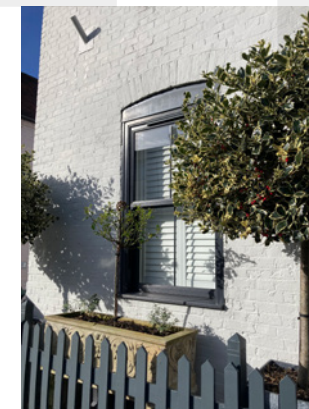
Example of replacement of a traditional window with uPVC unit.
