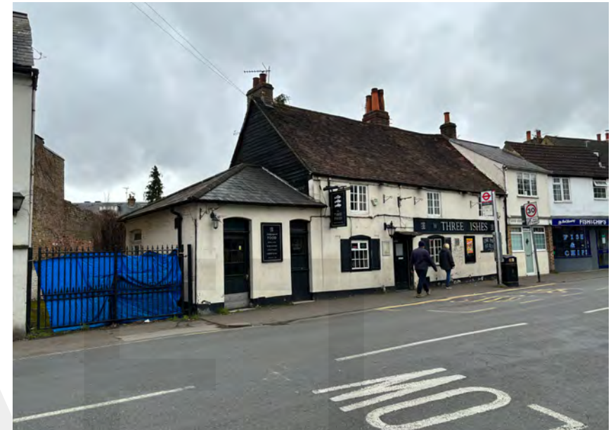
The Three Fishes on Green Street. The building is vacant and deteriorating. Damaged signage, failing paintwork and trailing wires depreciate the aesthetic interest both of the building and the wider streetscape.
