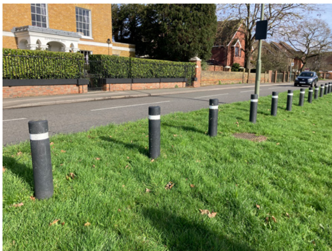
Modern bollards edging the village green detract from the historic character of the Conservation Area.
