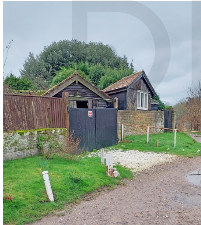
Former boathouses fronting onto Thames Side
