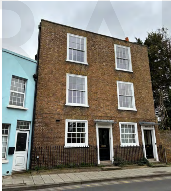
Riverside Cottage, Thames Street - a Georgian residence of some status with a restrained Neo-Classical façade.
