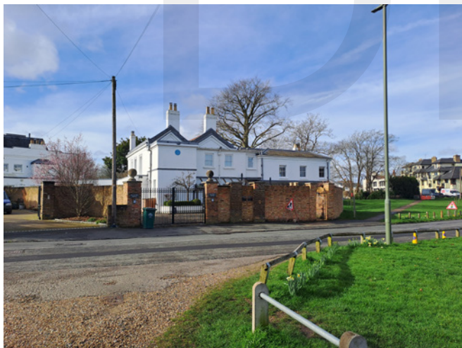
Examples of the prominent modern telegraph poles and street lights, these are in front of Peacock House and Halliford House on Walton Lane.
