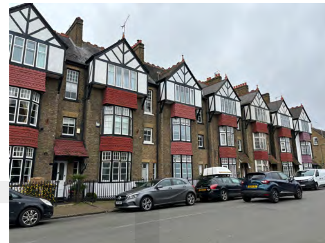
This late 19th-century terrace on The Avenue illustrates contemporary tastes for vernacular architecture, featuring false timber framing to the street-fronting gables and richly coloured hung tiles to the oriel windows.
