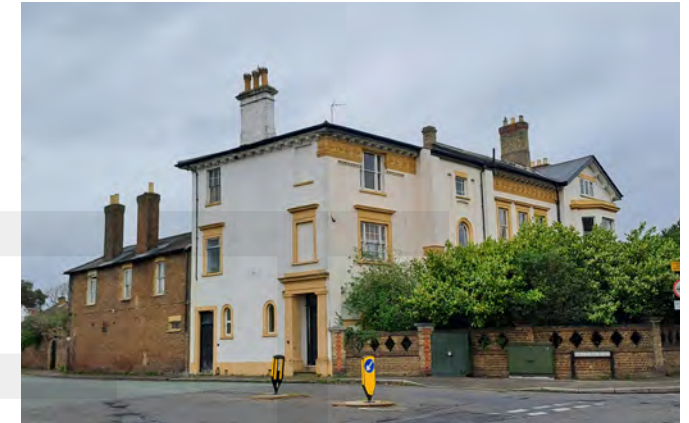
The 19th-century Weir House, which sits on the western boundary of the Conservation Area. The moulded eaves cornice and highly decorative terracotta frieze announce this as a high-status riverside dwelling.
