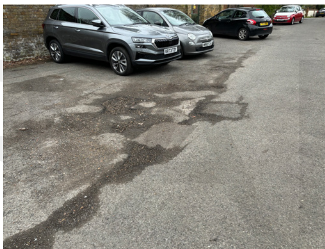
Potholed and uneven road surfaces detract from the visual appearance of the Conservation Area.
