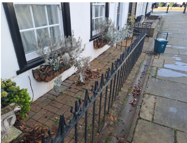
Traditionally styled cast-iron railings on Church Square.
