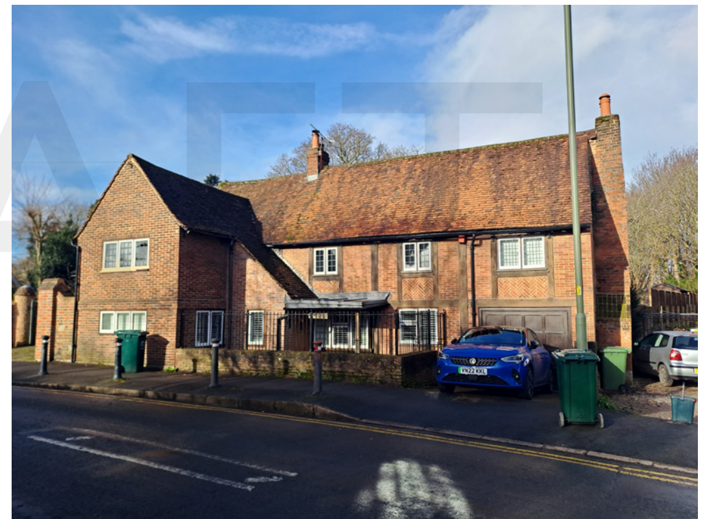
The Grade II listed Winches Cottage on Church Road, a vernacular building with a late 16th-century timber-framed core clad in 17th-century brick.
