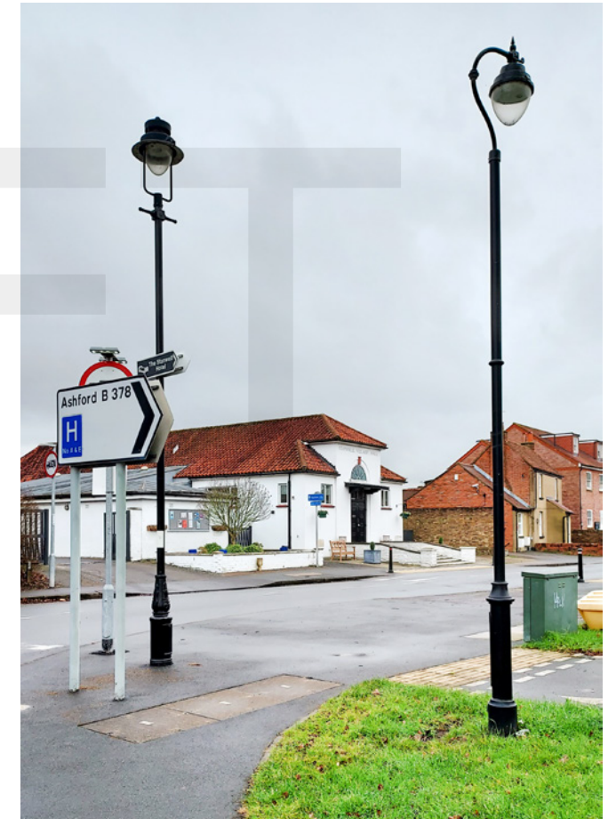
Examples of the traditional streetlighting in the Conservation Area.
