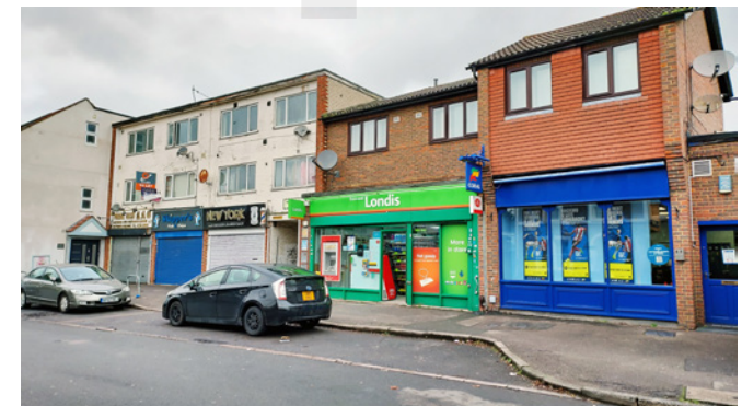
Modern shopfronts, which are out of keeping with the character of the Conservation Area
