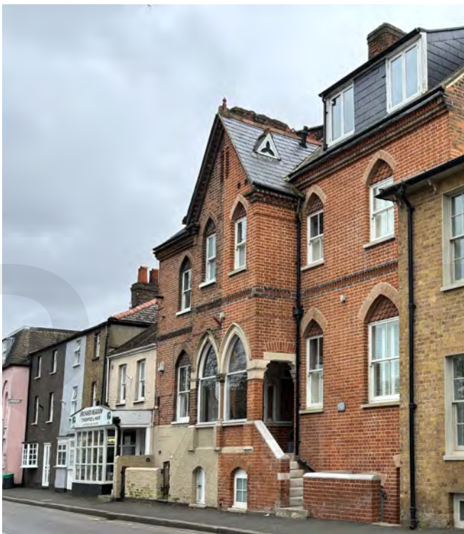
Thames Street are a pair of Victorian Gothic Revival houses incorporating a large street-fronting gable with trefoil-shaped vents and prominent pointed arches, articulated with red creasing tiles. The principal façade features richly coloured hung tiles and brick.
