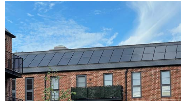
Flush photovoltaic panels incorporated into a roof
