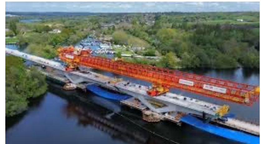
2.1 miles HS2 Colne Valley viaduct, each pre-cast span 80m, constructed with 700 tonne launching girder shipped from Hong Kong and assembled on site
