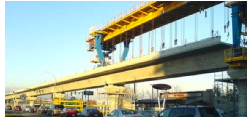
Launching girder construction technique - Submission to ORR Inquiry on Charging Framework for Heathrow, LARTS March 2016
