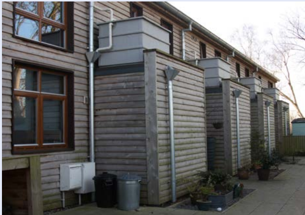
FIGURE 25: HOME RAINWATER CAPTURE SYSTEMS
