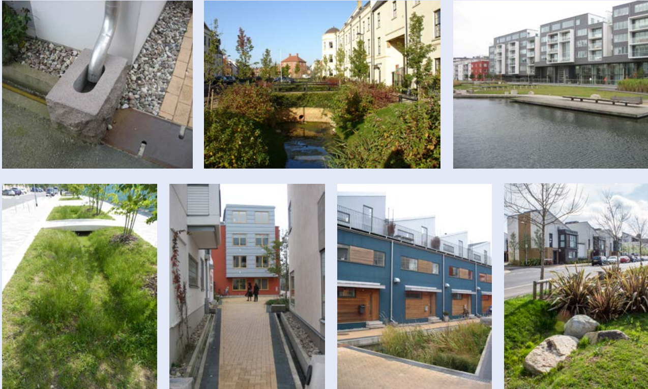
FIGURE 23: EXAMPLES OF SUSTAINABLE DRAINAGE SYSTEMS IN BUILT UP AREAS (TOP ROW: MALMO, SWEDEN; UPTON, NORTHAMPTON, HAMMARBY, SWEDEN) (BOTTOM ROW: CAMBRIDGE; MALMO, SWEDEN; MALMO, SWEDEN; NEWPORT)
