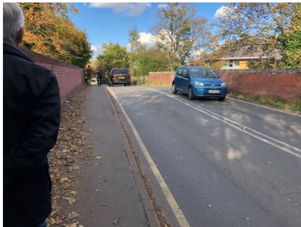
Figure 97. Pinch point at railway bridge on Green Street, with narrow carriageway and narrow footway on a single side.
