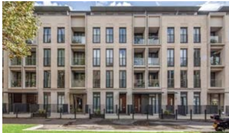
Figure 37: Portobello Square, London – regular ground-floor entrances and vertical articulation combine to make an attractive, fine-grain street (PRP)
