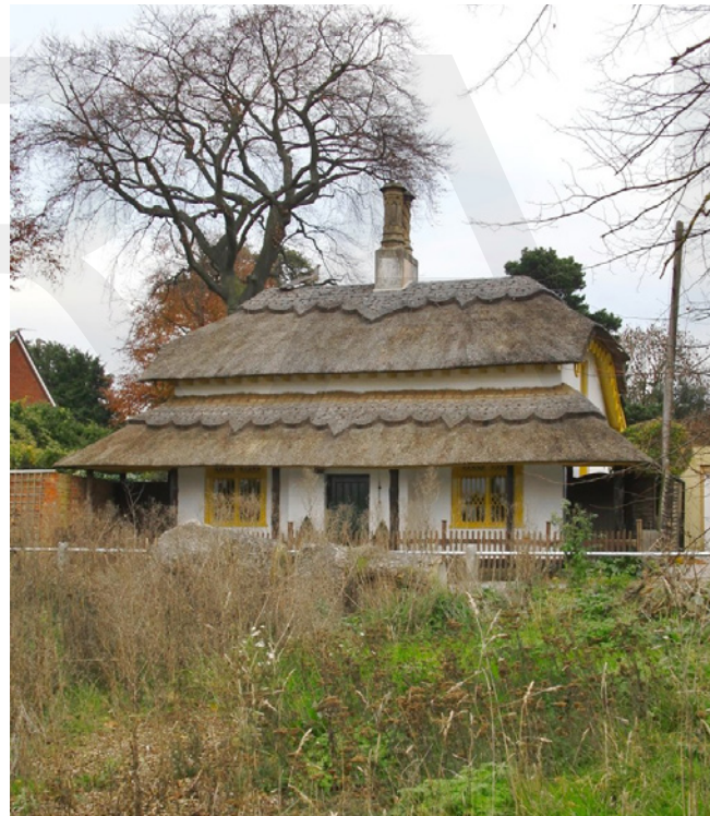
Thatched Cottage – a unique building type within the Conservation Area (Photo © Stefan Czapski (cc-by-sa/2.0))
