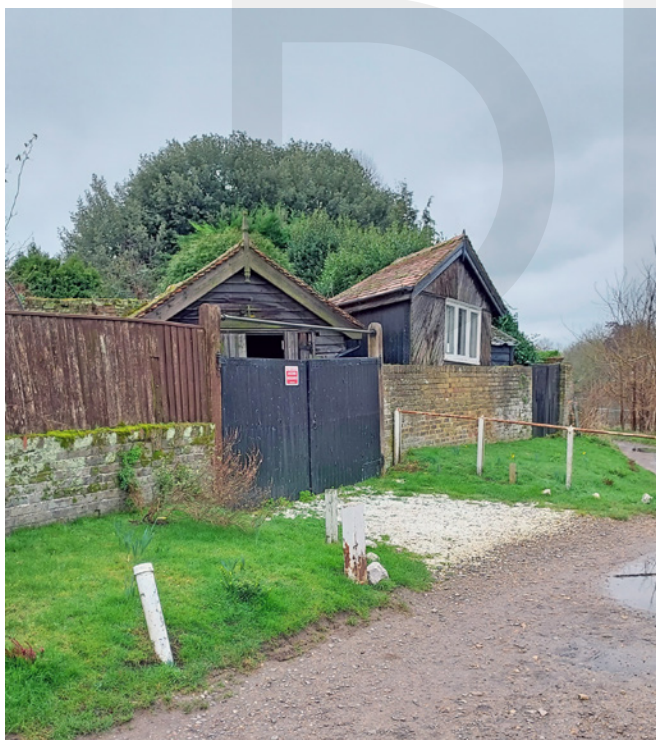
Former boathouses fronting onto Thames Side
