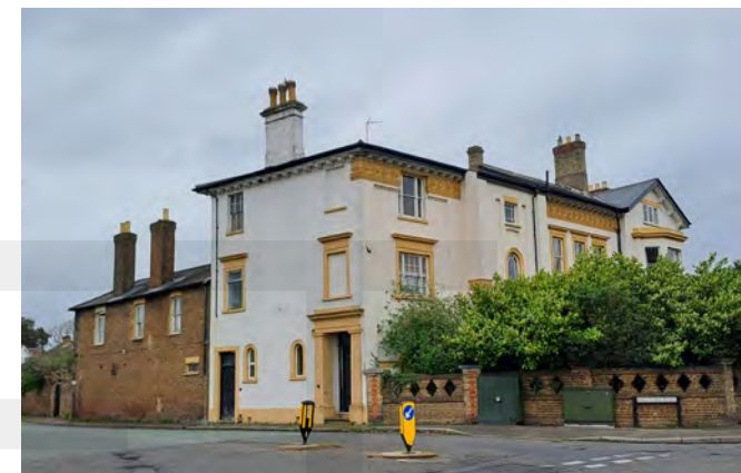
The 19th-century Weir House, which sits on the western boundary of the Conservation Area. The moulded eaves cornice and highly decorative terracotta frieze announce this as a high-status riverside dwelling.
