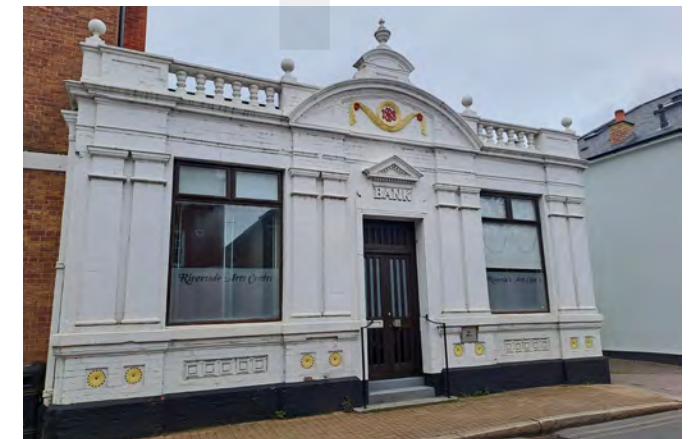
A late 19th-century Grade II listed bank on the north side of Thames Street. The ornate architectural treatment adds visual interest to the streetscape and the building illustrates the amenity value historically supported in this area of the village.
