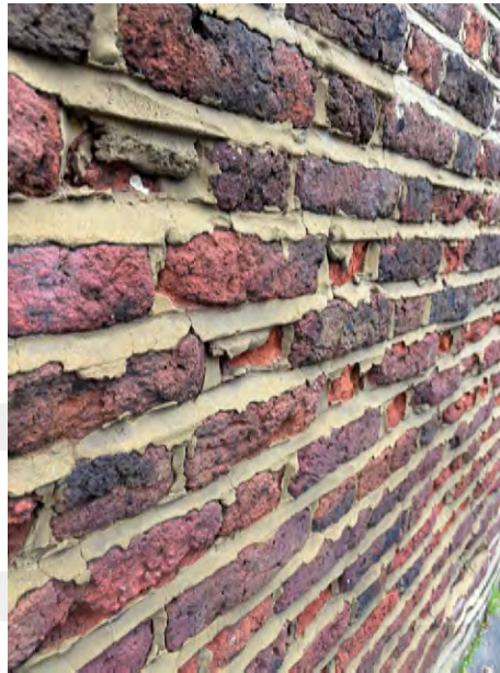
An example of ribbon pointing with cementitious mortar to a historic brick boundary wall in the Conservation Area.
