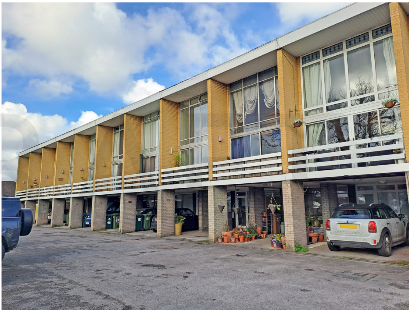
The south elevation of three-storey Modernist block in phase 1, to the north of the estate.
