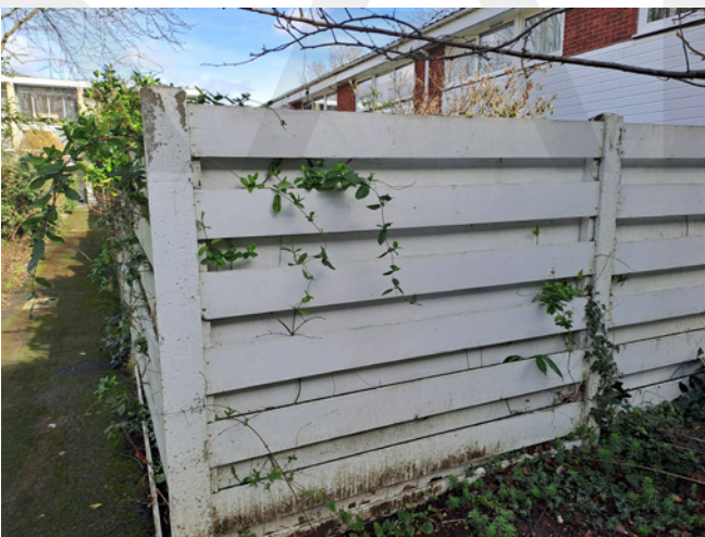
Plain, white-painted timber 'hit and miss' fencing in phase 3 of the estate.
