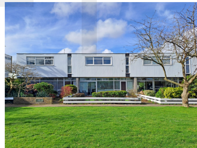
Many windows in the estate have been replaced with uPVC units as shown here at first floor level and in the central dwelling at ground floor.
