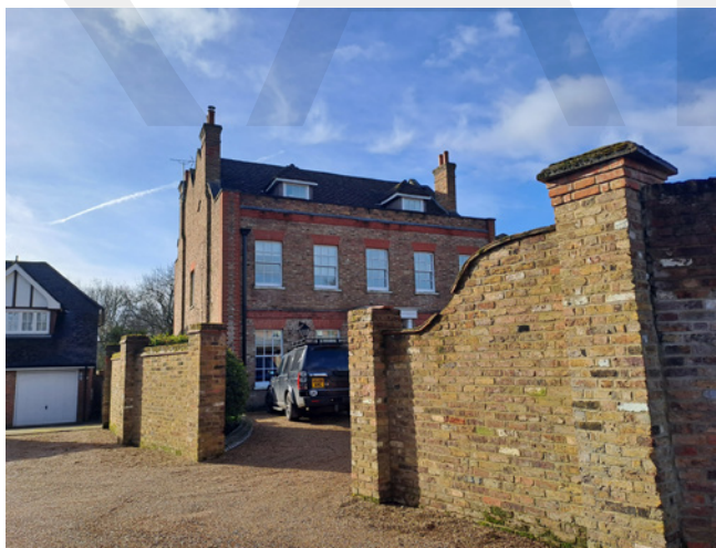
Millbrook House, Chertsey Road. This early 19th-century building utilises a restrained Neo-Classical style with a highly symmetrical façade, parapet, formal portico and flat arches over sash windows.
