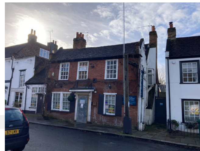
The Kings Head pub, currently vacant and in need of maintenance and repair
