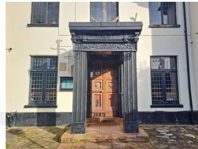
Classical motifs to the flat-roofed portico at the 19th-century Anchor Hotel on Church Square. The use of decorative moulding is unusually rich when compared to the restrained use of Classicism seen elsewhere in the Conservation Area. The age of the portico and its relationship to the original building is unclear, although it is visible in a photograph of the hotel from 1915. 02
