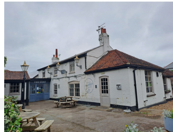
The Goat Inn, a historic complex with a mixture of single and double storey ranges, the oldest of which date from the 18th century.
