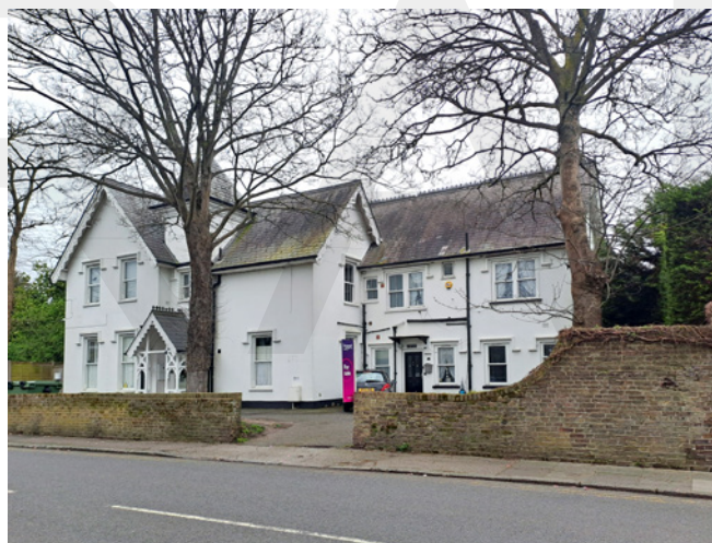
42 Upper Halliford Road, built between 1898 and 1912, illustrates the contemporary fashion for the Tudor Gothic style – with hood moulds over the windows, decorative barge boards, and a strong emphasis on verticality achieved through the steeply-pitched roofs and pointed arches to the front porch.
