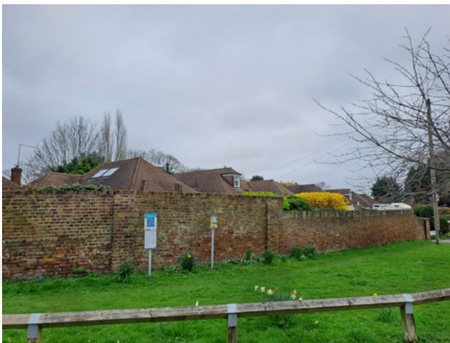
The brick wall separating nos. 1-8 Holmbank Drive from the village green, parts of which constitute the historic boundary wall of 42 Upper Halliford Road. The grounds of this large house were subdivided after 1934 to accommodate additional residential development along the northern side of the green.
