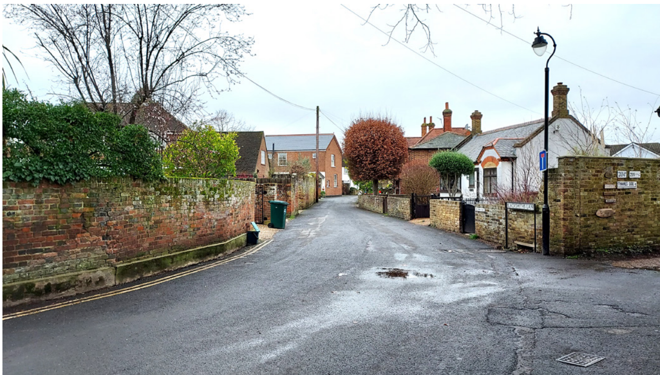
The entrance to Blacksmith’s Lane, where the informality of the highway and boundary walls emphasise its access-only character. Also note the traditional street lantern.
