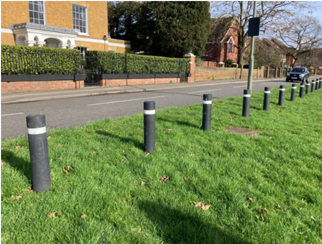
Modern bollards edging the village green detract from the historic character of the Conservation Area.
