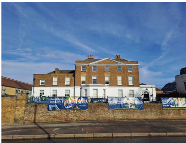
Halliford School, originally built as a house in the late 18th-century. The building is typically Georgian in its use of restrained Neo-Classical decoration, with symmetrically arranged sash windows under flat arches, a plain eaves cornice, a simple pediment, and a parapet.
