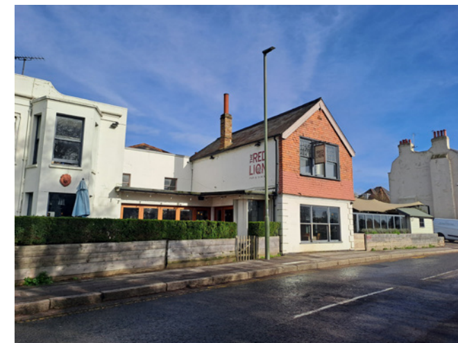
Hung clay tiles to a street-fronting elevation at the Red Lion, Russell Road.
