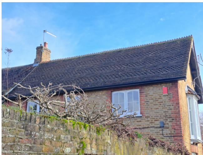
Decorative clay tiles to the roof of the Grade II listed Thamesfield Cottage on Russell Road.
