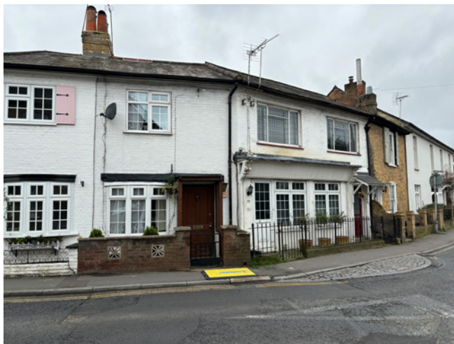
Historic properties at the south of the character area, adjacent to the historic core. Note the redundant fascia board which denotes a former shopfront, since lost.
