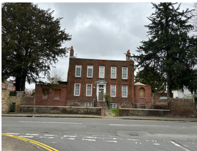
106 French Street, an early 18th-century dwelling on the corner of French Street and The Pennards. The deep front garden creates a strong sense of separation from the public highway and adds to the open character of the road in this area. The principal façade is framed by mature trees.
