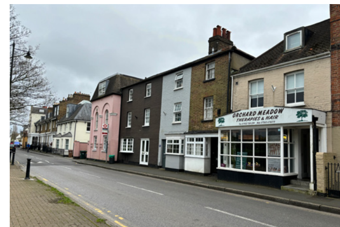
The south side of Thames Street, opposite Sunbury Park. The variation in colour, materiality, height, and usage of the buildings creates a lively street scene.
