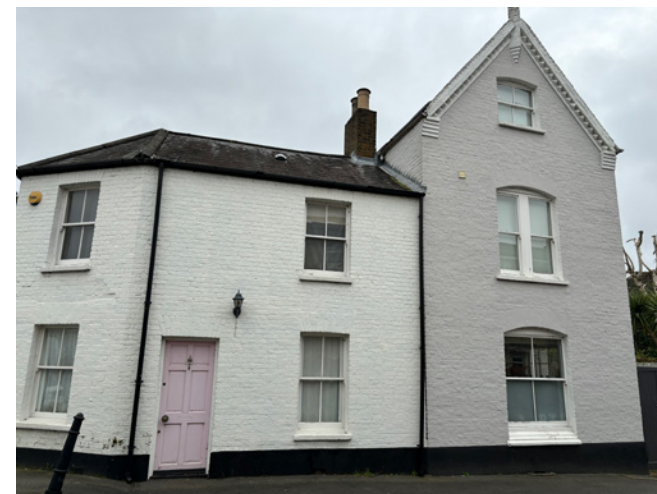
The steeply pitched roof and large street-facing gable end to No. 6 Green Street is typical of later 19th-century domestic architecture.
