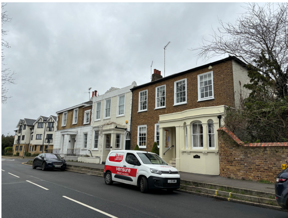
Contact House, Rivercote and Willowbank, a terrace of Grade II listed 18th and early 19th-century riverside residences on the corner of Thames Street and French Street.
