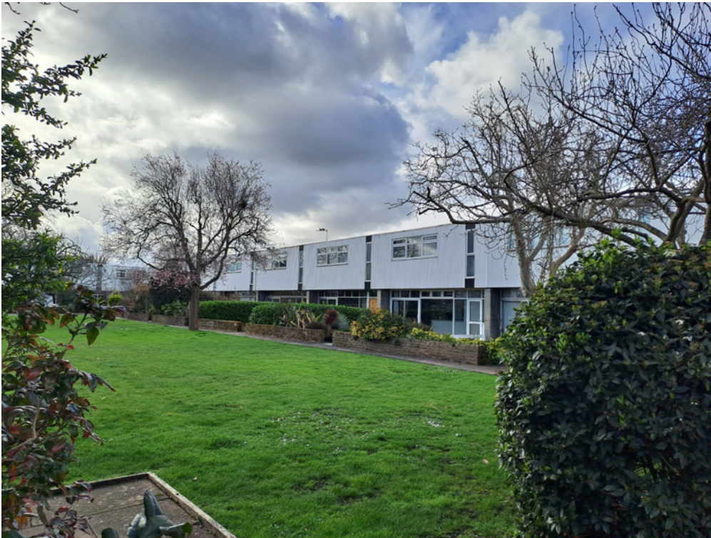
Oblique views of the linear blocks and across the green spaces are a key part of experiencing the estate.
