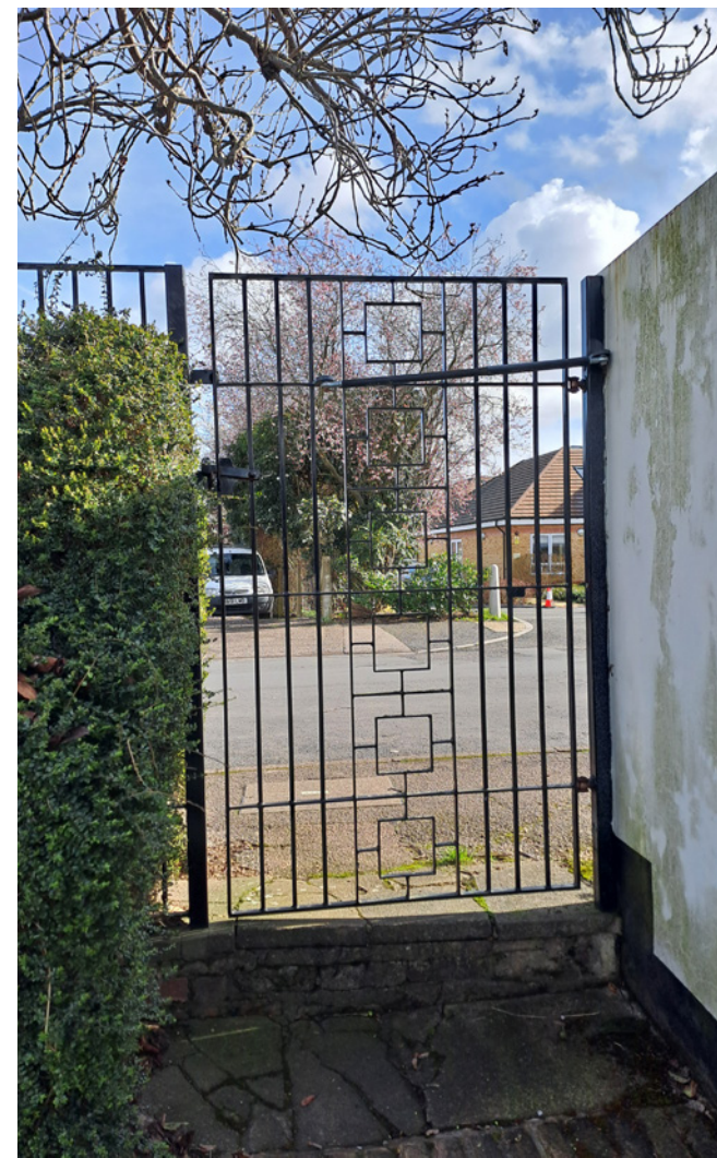
A sympathetic example of a gate which utilises clean, geometric lines and complements the Modernist character of the wider estate.
