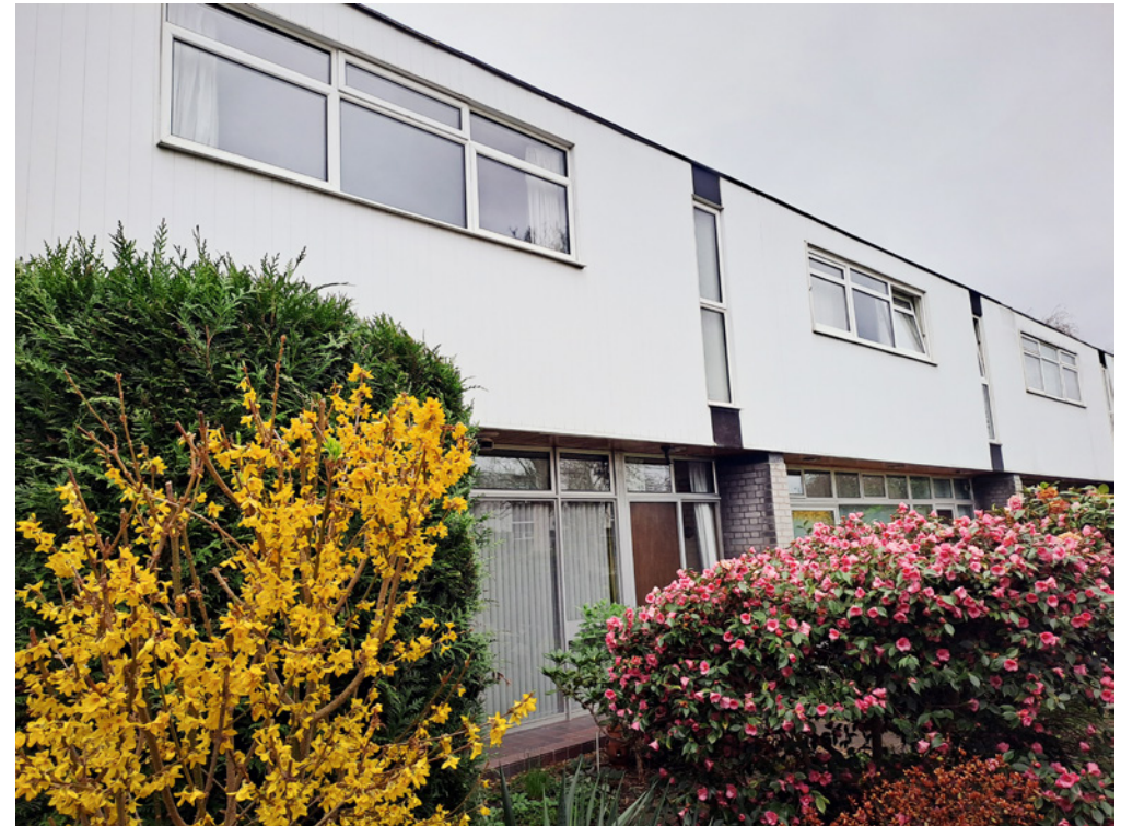
Modernist terraces in phase 2. Note the horizontally-configured windows and projecting upper storey.
