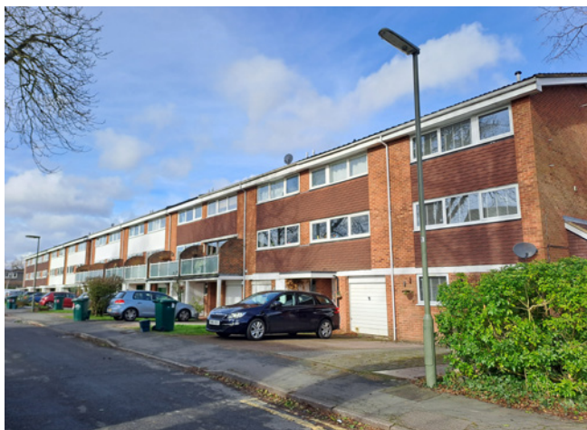
The southern-most terrace on the estate, part of phase 3. The approach is far less austere than phases 1 and 2, incorporating a warmer materials palette and decorative hung tiles.
