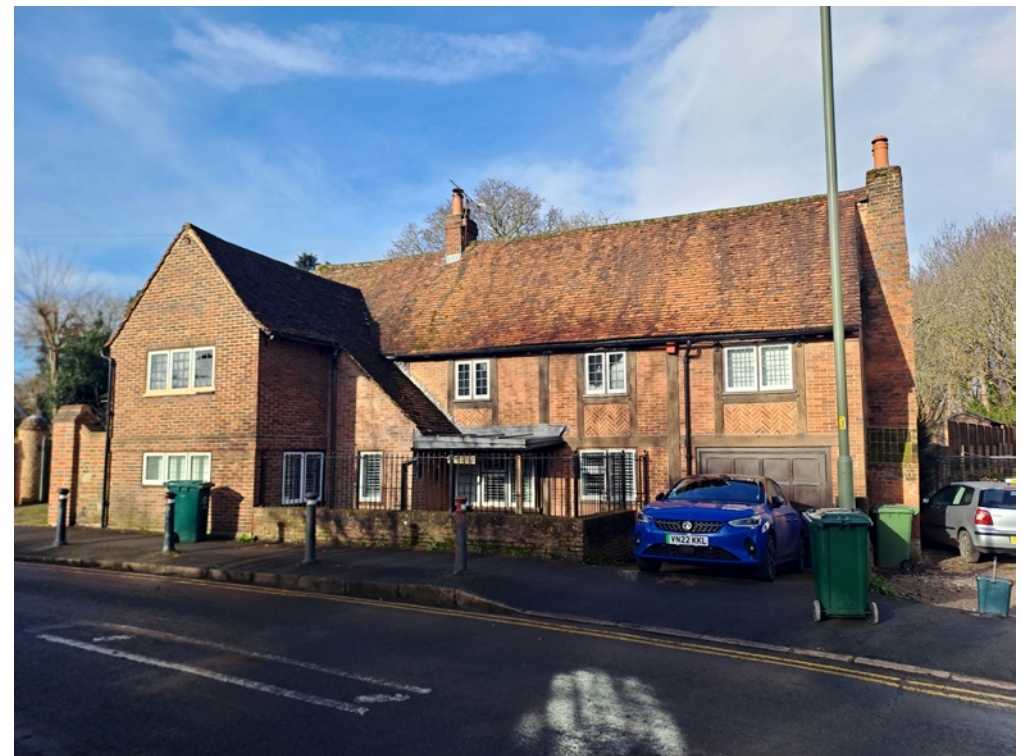
The Grade II listed Winches Cottage on Church Road, a vernacular building with a late 16th-century timber-framed core clad in 17th-century brick.
