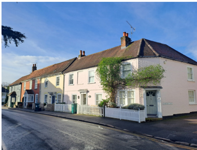
A terrace of Grade II listed 18th-century houses on Church Road. Typical 18th-century features include the regular arrangement of sash windows, small flat-roofed porches supported by scrolled brackets and dentils under the eaves (to No. 2 Lime Tree Cottages).
