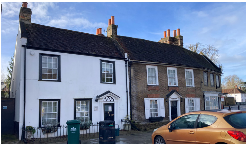
Historic timber-framed sash windows to the 18th century buildings on the south side of Church Square.
