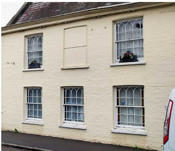
Unusual Gothic windows on Oak Road
