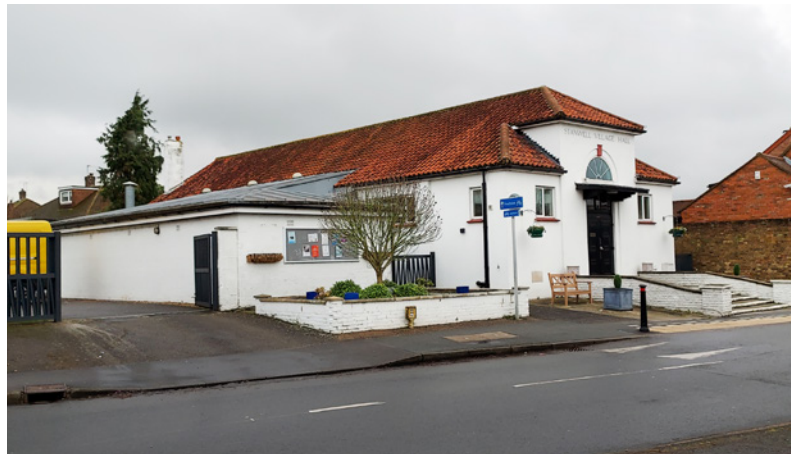
The village hall on the High Street.
