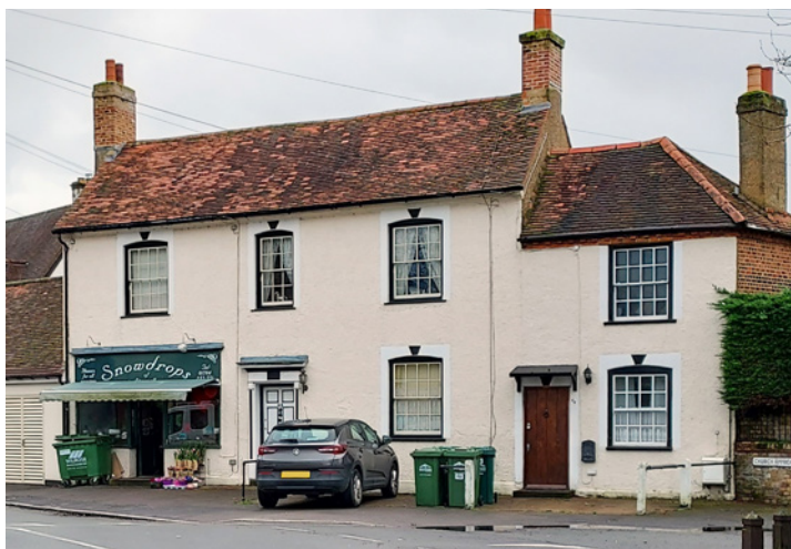
Traditional timber sash windows on the High Street
