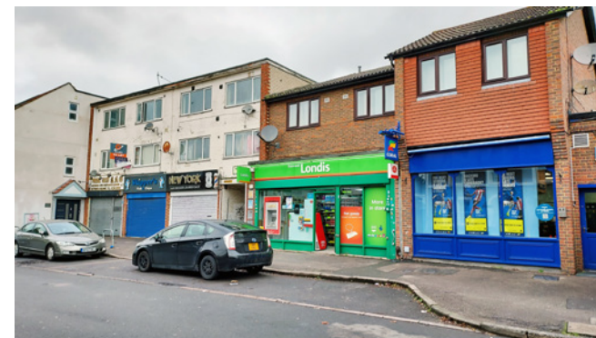
Modern shopfronts, which are out of keeping with the character of the Conservation Area
