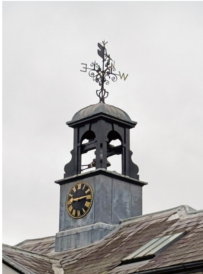
The distinctive lead-covered cupola on Clock Cottage, Halliford Road.
