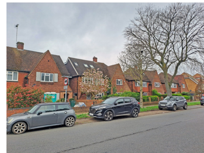
Four pairs of mid-20th century houses on the west side of Upper Halliford Road. The influence of the Arts and Crafts movement can be seen in the asymmetrical roofline, leaded lights, use of richly coloured red brick and decorative hung tiles.
