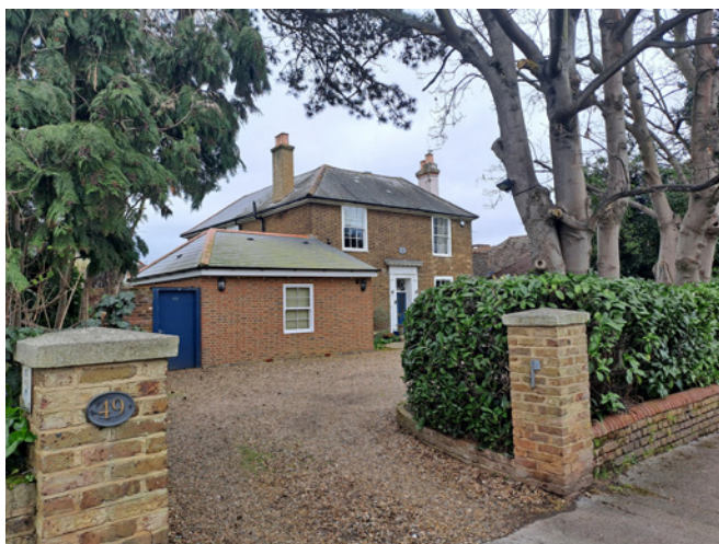
49 Upper Halliford Road. An 18th or early 19th-century dwelling with typical Georgian detailing including a square plan, regularly arranged sash windows and a small portico articulating the principal entrance.
