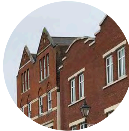
Gable end roof forms
