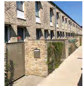
Integrated bin and cycle storage
