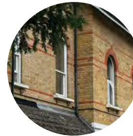
Changes in brickwork
