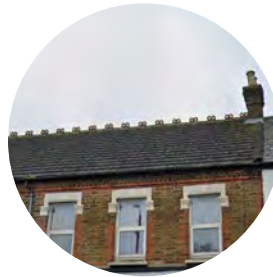
Roof line features
