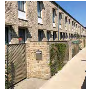
Integrated bin and cycle storage
