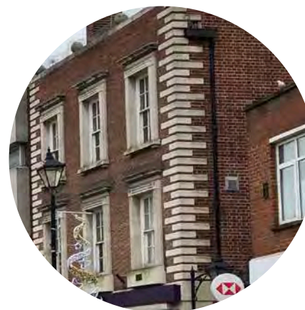
Corner brickwork detailing and brick variation
