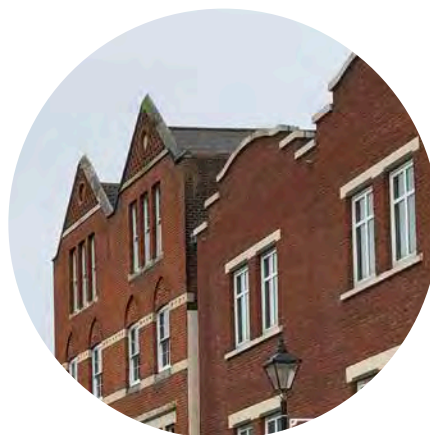
Gable end roof forms
