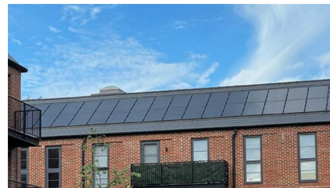
Flush photovoltaic panels incorporated into a roof
