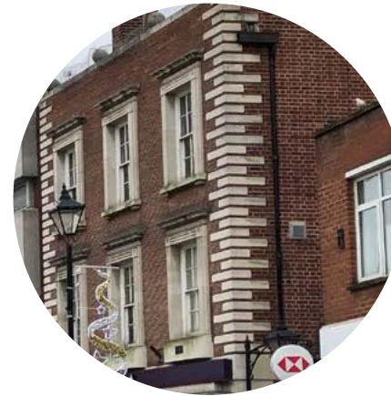
Corner brickwork detailing and brick variation
